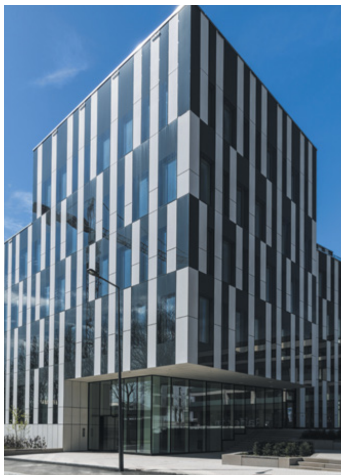
Immeuble "Le White Pearl"
